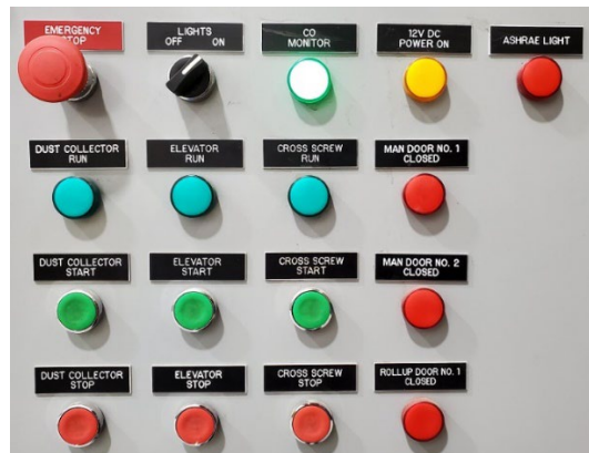
ABS – Below Floor Sweep in Recovery Blast Room control panel and warning decals
