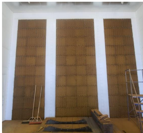
CFS Paint Booth – Filter System
