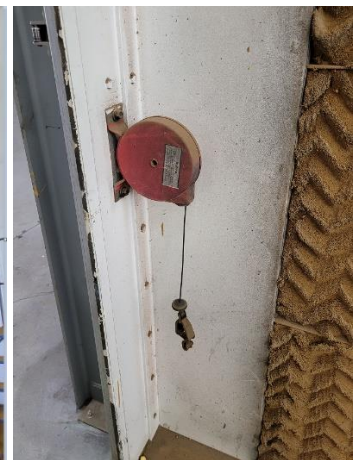
Ground cable - CFS Paint Booth
